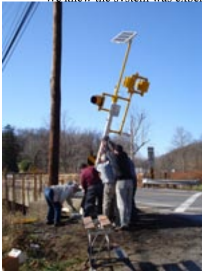
Volunteers raise one of the units on Cliff Mine Road. Charlie Beaumariage measures while Tim Killmeyer, Dennis Pfeiffer, Jack Peth and Bob Teachout raise the unit. Photo by Janet Shaffer
