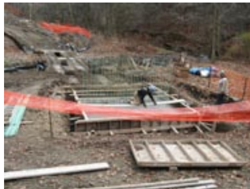
The Piney Fork Bridge site on November 10, 2008. The temporary fence in the foreground surrounds the west abutment foundation slab poured a short time before. Reinforcing steel to tie the foundation to the abutment concrete can be seen standing in the photo. Mats were placed over the concrete to insulate it and prevent freezing after the photo was taken. The abutment pour was scheduled for November 12. The temporary fence in the background is around the hole dug for the caissons of the east abutment.
